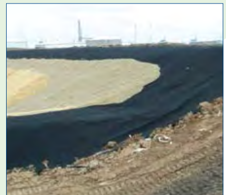
A typical hazardous landfill cell lining under construction
