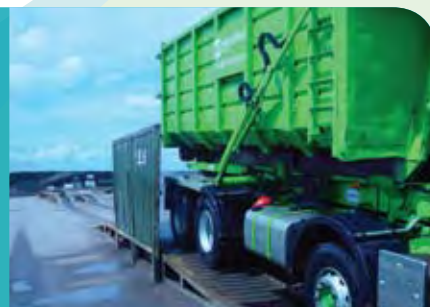
A lorry completes wheel washing before leaving the site
