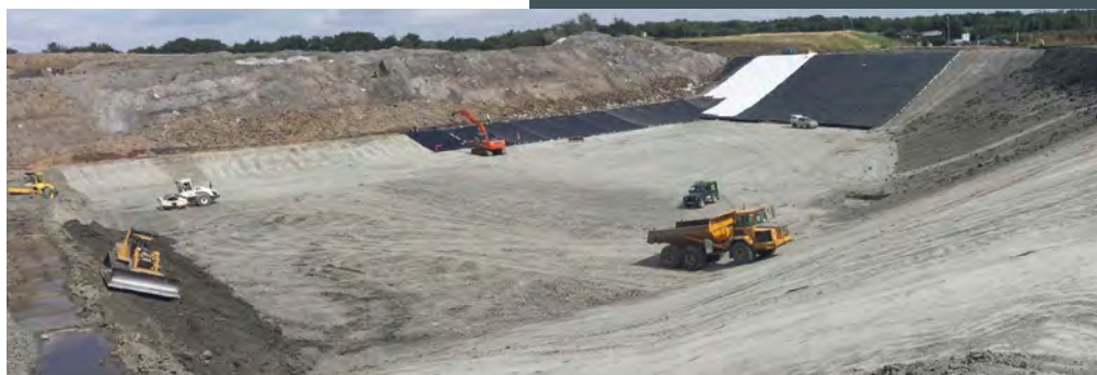
Landfill cell being engineered
