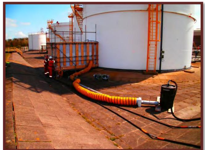
Figure 1: Ventilation Set-Up for Inert Tank Entry Clean
